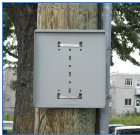
Figure 14, Pole bracket banded to utility pole
