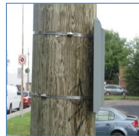
Figure 16, Profile view of pole bracket
