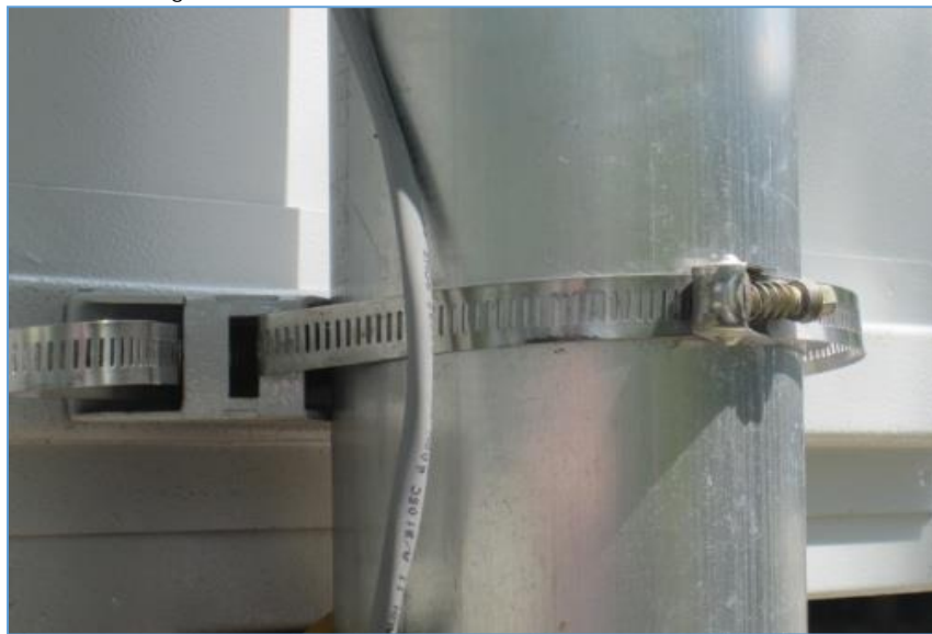
Figure 5, Sign Secured to a Pole with Banding Strap
